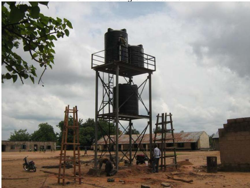
Pic. 10: Tower completed with 14,000 litres capacity tanks Mounted
