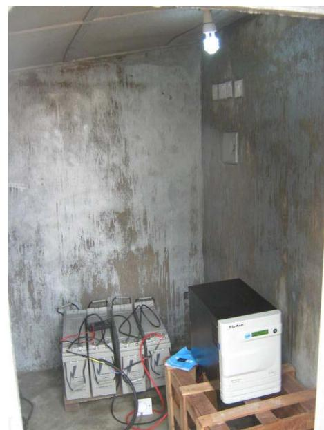
Pic. 17: Inverter with batteries powering a lamp
